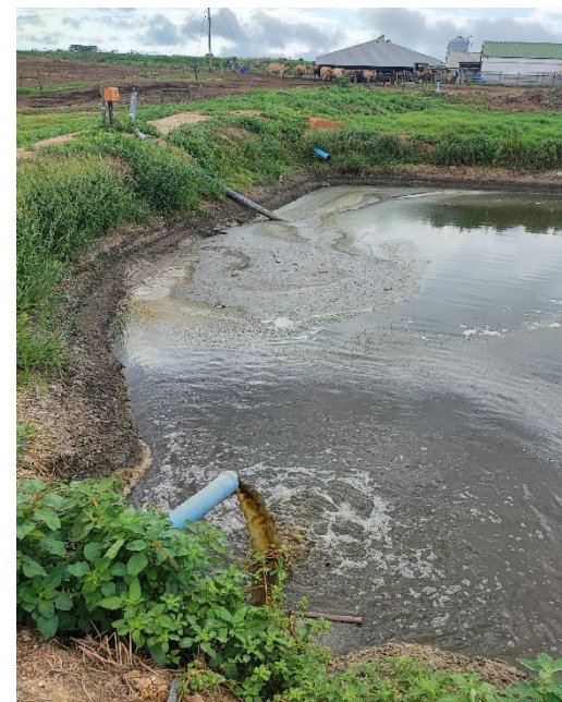
A typical effluent storage pond.
