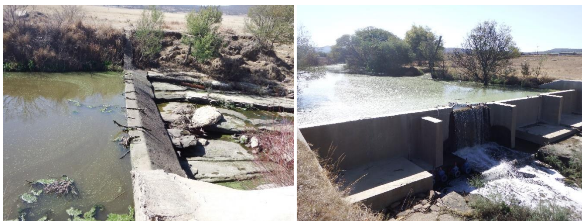
Figure 9. Water abstraction points above instream weirs showing reduced base flow downstream during low rainfall season (summer rainfall area, Kwa-Zulu Natal). Water quality upstream has obviously high suspended sediment and algal growth, and barriers restrict upstream movement of aquatic biota.
