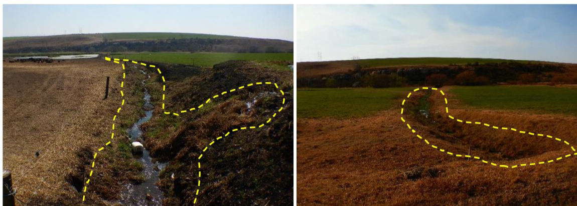
Figure 33. Examples of linear drains on the KZN farm site.
